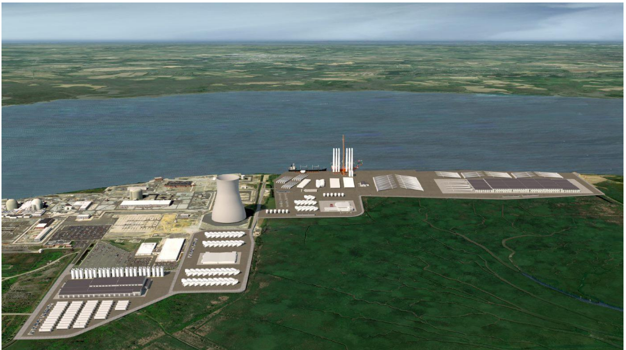
Overhead of New Jersey Wind Port being built on Delaware Bay in Lower Alloways Creek.
